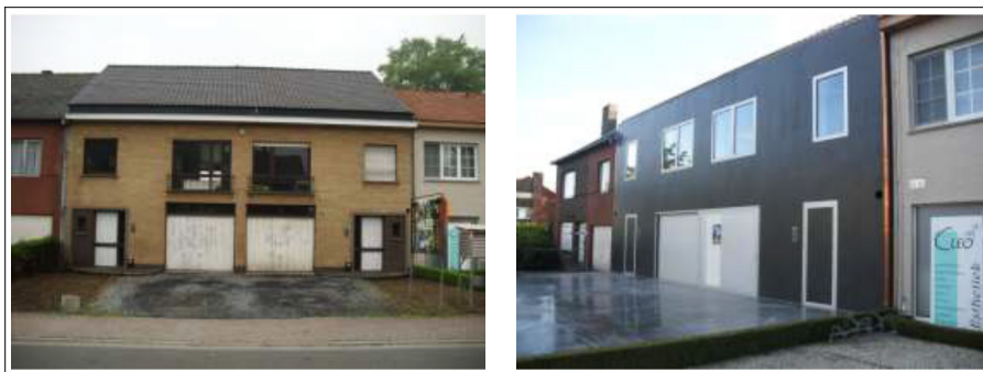
Retrofit of 2 row houses from the 1970s. Before (left) and after (right) © Benergie.be - Architect L. Dedeyne
