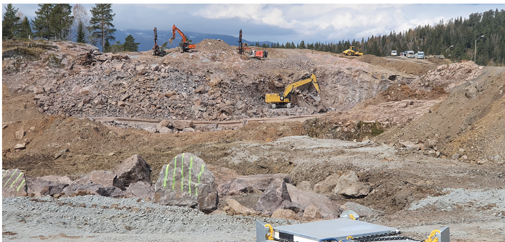
Figure 5 Excavation for the new E18 highway from Sandvika to Hønefoss at Sollihøgda.
