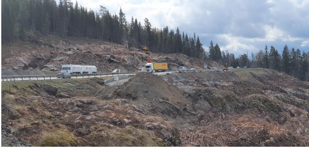
Figure 2 Preparation for drilling and blasting during tunnel construction project on the new E18 highway from Sandvika to Hønefoss at Sollihøgda.
