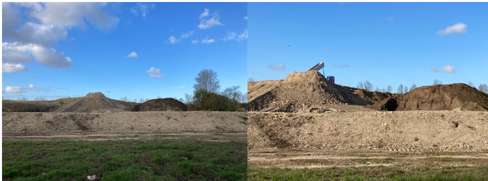
Figure 1 Use of unpolluted and slightly polluted surplus soil in a nature and landscape project near Copenhagen.
