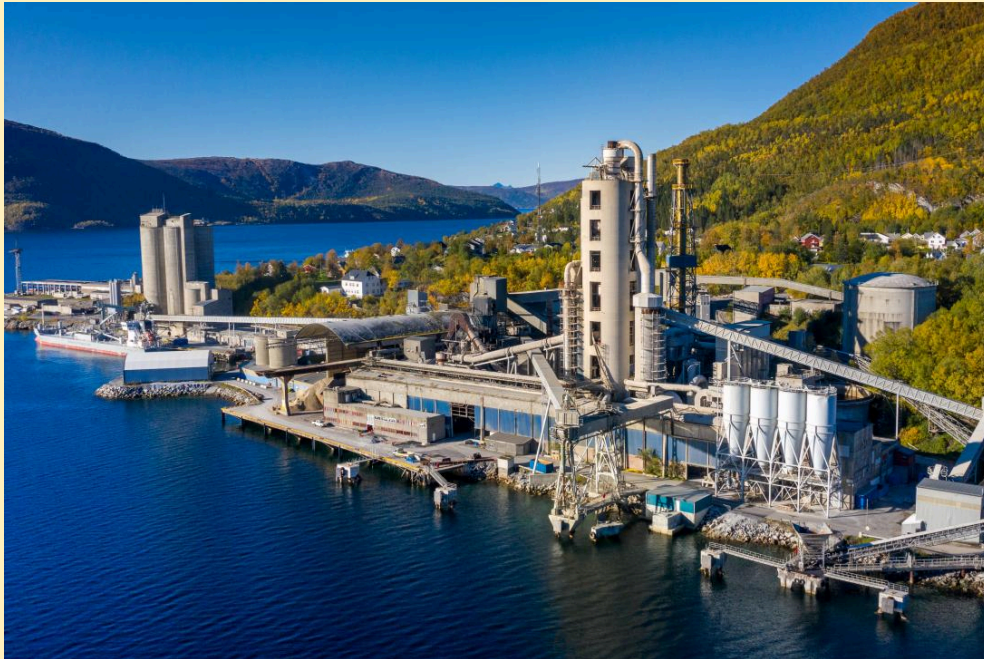
Norcem AS Kjøpsvik cement plant
