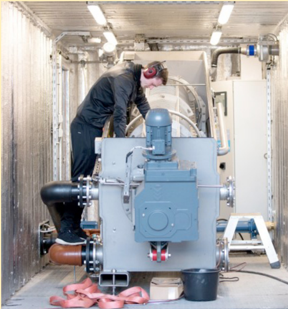
A technician works on a Blue Ocean Technology screw press
