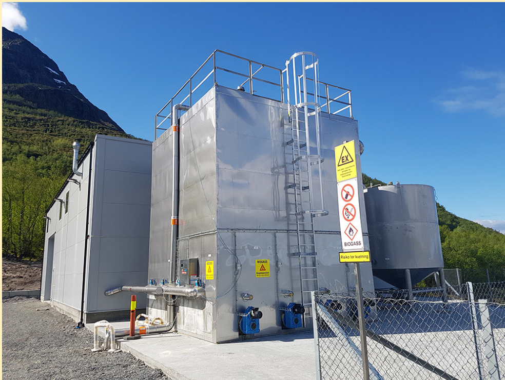
Photo of a Sterner Biogas reactor on a fish farm
