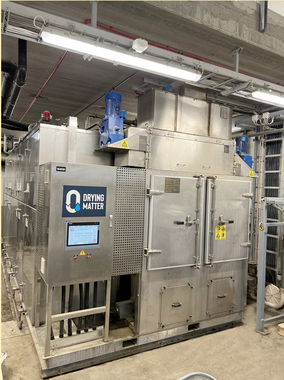
A Drying Matter heat pump sludge dryer
