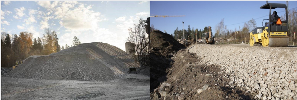
Intermediate storage of reclaimed concrete (left), use in road base (right).
