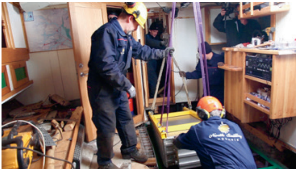
Figure 3. Installation of one of the batteries under the floor in Opal.
