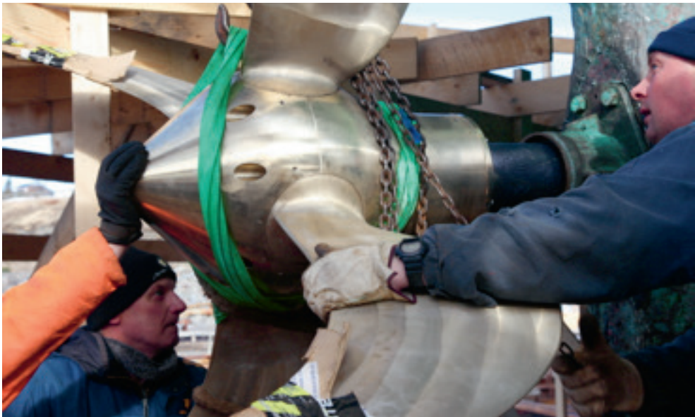
Figure 5. Installation of the propeller into Opal. The blades are in the flat sailing position.
