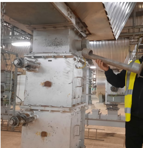
Figure 3.29. Sampling hole and sampling rod at ARGO's MSWI facility (A). A view of several FA precipitation stages connected to a conveyor belt line on the bottom (B). All stages were sampled during the project. Photos: ARGO.
